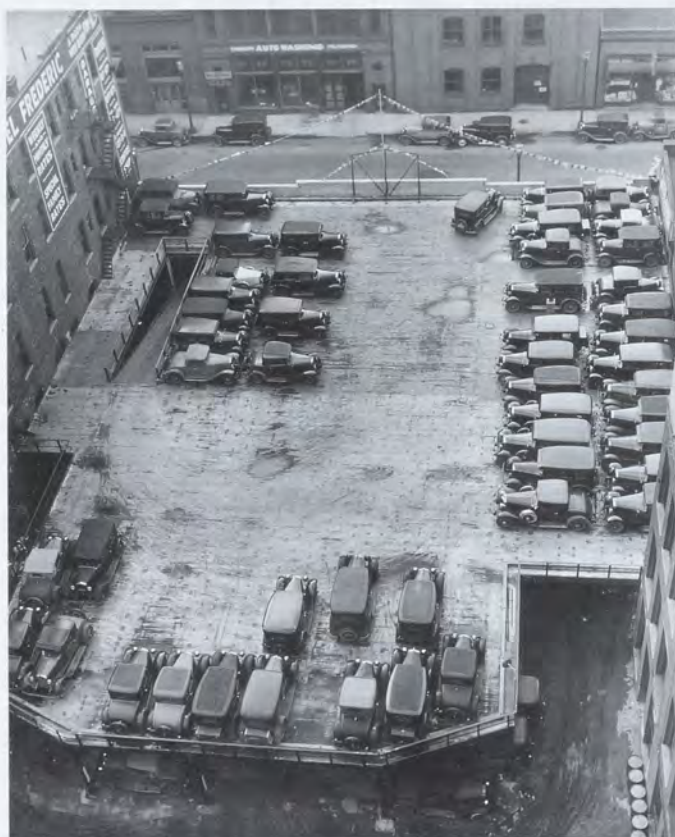
DeLoop Service Station and Parking Ramp 384 Cedar c. 1931. A garage built in 1905 was torn down for a filling station in 1928. Three years later the 100 x 130-foot parking roof was added. Photograph by Peter Schawang.
