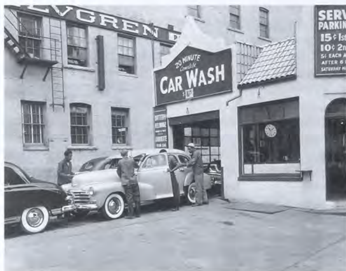
In 1949, Harry Schloff wisely located across from the Emporium Department Store. It was primarily for short-term parking but, like other such businesses, gained additional income by adding complementary services.
