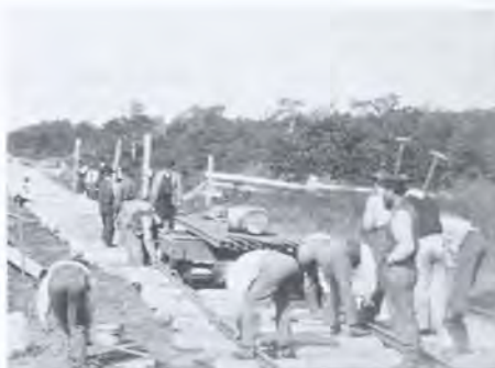
A track crew, probably working for the St. Paul & Pacific, laying rails in a westerly direction from St. Anthony toward Anoka about 1865. Benjamin Franklin Upton stereographic photo. Photo courtesy of the Minnesota Historical Society.
