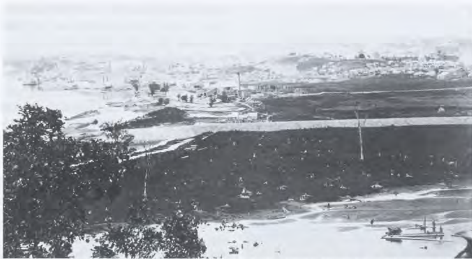
St. Paul from Dayton's Bluff looking west about 1861. Clearly visible as a white horizontal line is the 1,400-foot track that had been graded and laid across the marsh below the bluff. In the lower foreground there are stumps, the remnants of a maple forest formerly used by the Dakota for sugar making each spring. At the far left, hundreds of ties are stacked up awaiting construction. Benjamin Franklin Upton photo. Photo courtesy of the Minnesota Historical Society.
