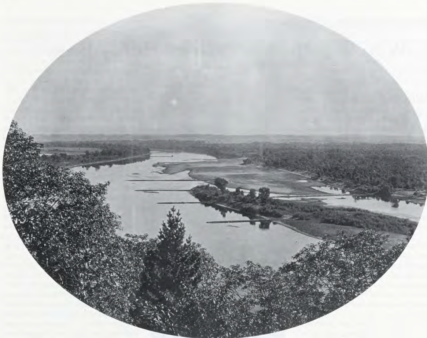
Wing dams along the Mississippi at Pine Bend. The dams deflected the current to the main channel, while eddies behind the dams trapped sediment. Over time, these forces narrowed and deepened the river.
