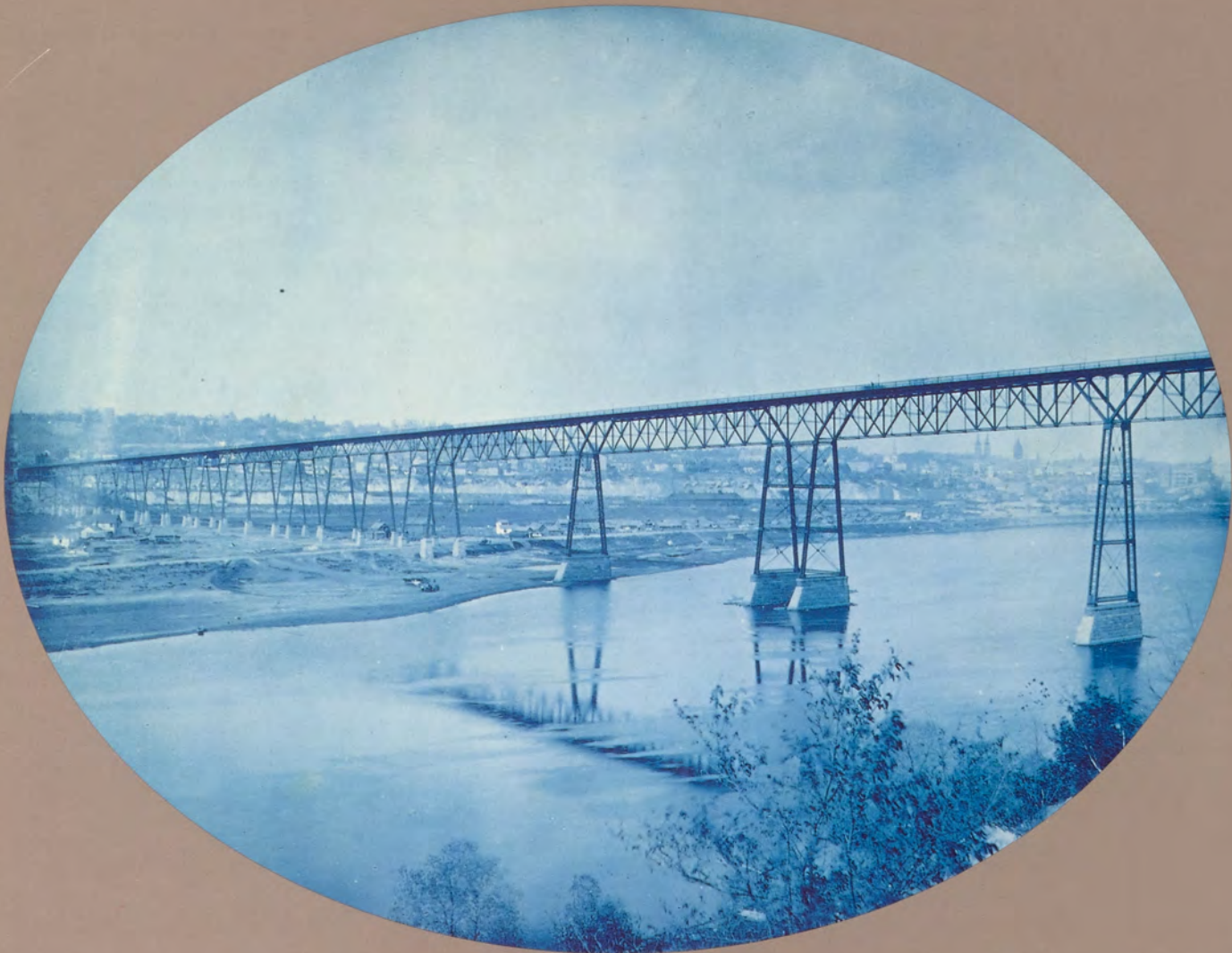
Henry Bosse's photograph of St. Paul's old High Bridge after it opened to horse-and-buggy traffic in 1889. Because the bridge offered easy access to the Cherokee Heights neighborhood, settlement of this section of the West Side began in earnest. A modern bridge replaced the old bridge in 1985. See article beginning on page 4. Photograph from the St. Paul District, United States Corps of Engineers.
