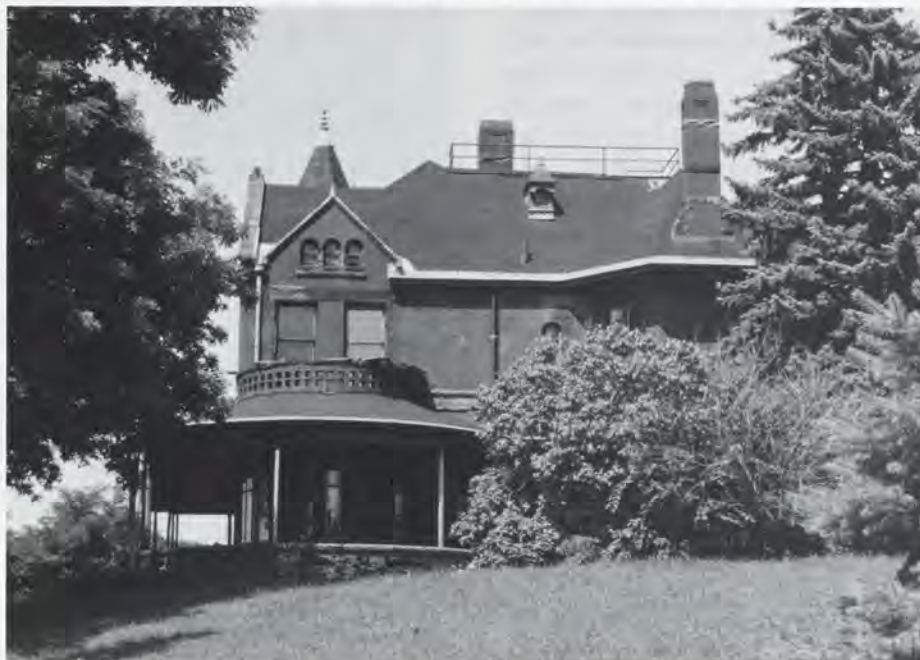
The house Peter and Marie Giesen built in the fashionable Dayton's Bluff neighborhood, home to a large community of St. Paul's German-Americans. The house still stands. Photo from the author.
