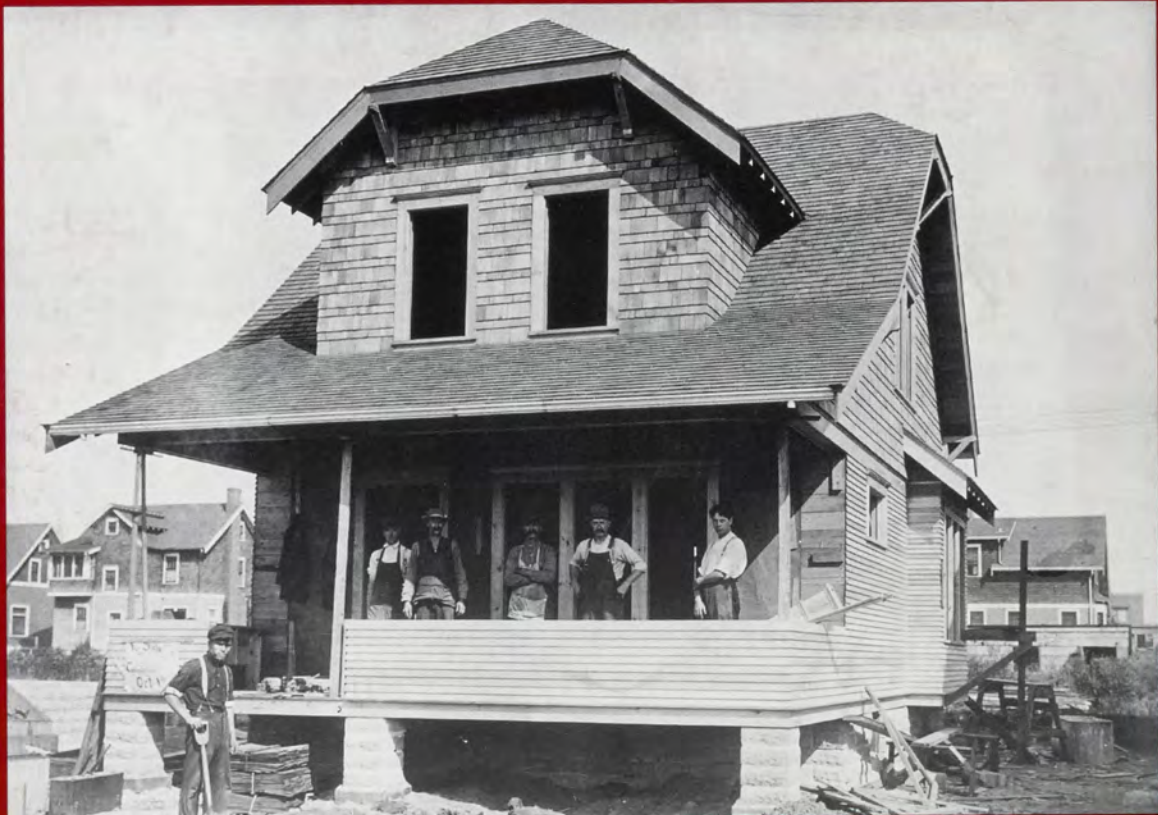
Easy to build. This is a partially finished bungalow in St. Paul in 1906. Minnesota Historical Society photo. For more about the bungalow craze of the early years of this century, see page 15.
