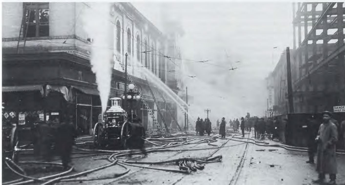
The great St. Paul Public Library fire, April 27-28, 1915. The building housed the city's second Market House, as well as the state legislature for a time after the second state Capitol burned down. Minnesota Historical Society photo.
