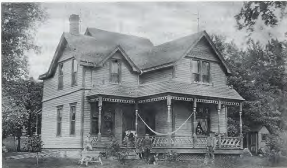
The Stacy home in St. Paul Park, with the elder Stacy at the far right. Walter stands stiffly in the front center. The girl on the left is not identified. Mrs. Stacy lounges on the porch.
