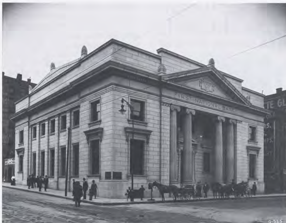
The First National Bank building at Fourth and Minnesota in 1908.
