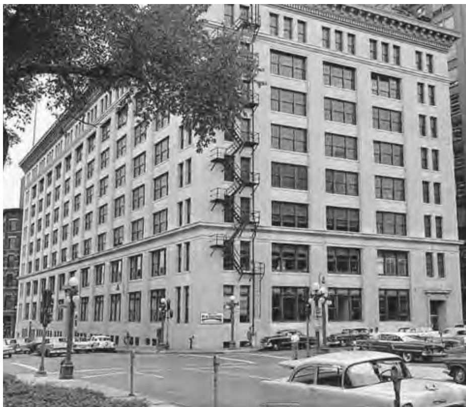
The Nalpak building at 333 Sibley in 1959, as seen from Mears Park. Note the fire escape and the absence of the main entrance on East Fifth Street. Owned at the time by John J. Kaplan, president and treasurer of the Globe Paper Box Manufacturing Company of St. Paul, its name was changed to the Nalpak Building (Kaplan in reverse).
