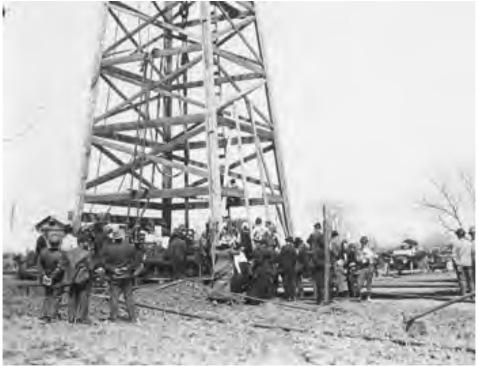
The well (top) that Lario Oil & Gas drilled on the Wenrich lease in 1928 drew a crowd of on-lookers. This well was not only an outstanding producer, it was also the first well ever drilled in Kansas using a hydraulic rotary system (below) instead of the older cable tool rig. Cable rigs were less expensive than rotary rigs, but rotaries typically drilled faster and to greater depths. Photo reproduced by permission from the private collection of the Lario Oil & Gas Company.
