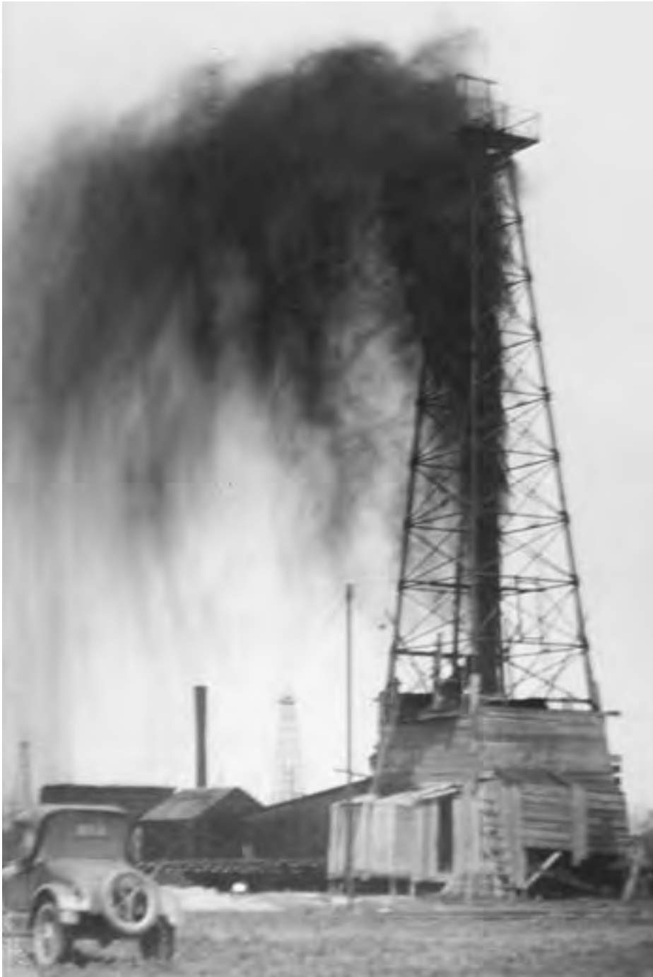
Lario Oil & Gas Company drilled this gusher on the Wenrich lease in the Oxford Pool in Sumner County, Kansas. The photograph was taken on April 15, 1928. This well yielded Lario's first oil production and marked its beginning as a successful oil prospecting company. The Wenrich lease is still producing today. Photo reproduced by permission from the private collection of the Lario Oil & Gas Company.
