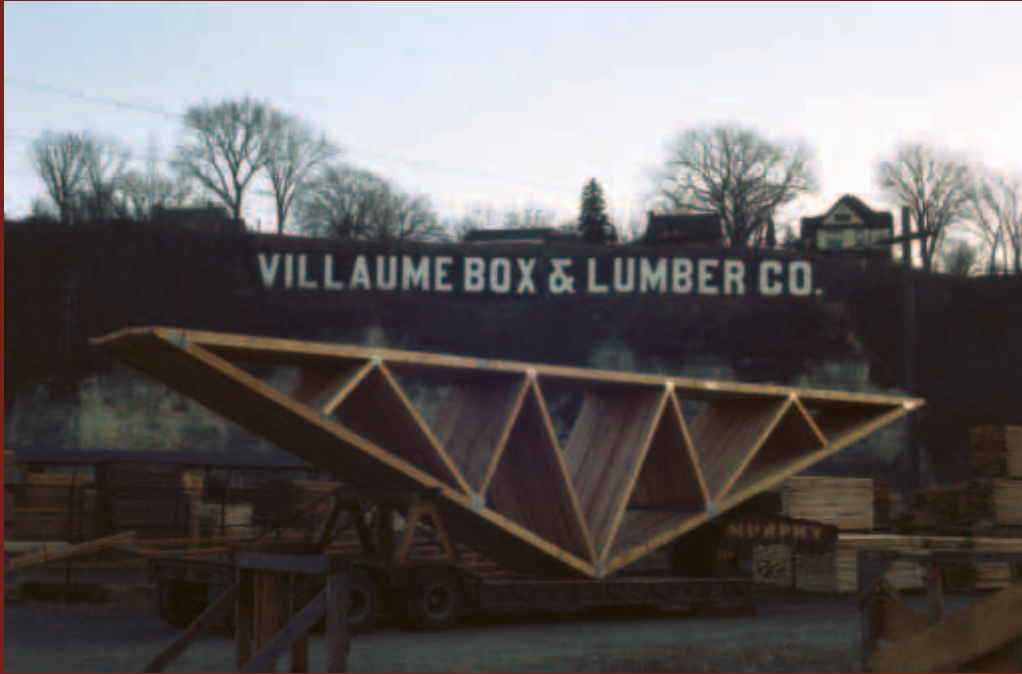
This late-afternoon photograph taken in the 1960s shows a supply of building trusses with their "Gizmo Gussetts," or metal connector plates, ready for shipping on a Murphy Trucking Company flatbed trailer in the yard at Villaume Box & Lumber Company. In the background is the Villaume sign, complete with hundreds of light bulbs, mounted on the bluffs on the West Side. Various residences are just visible beyond the sign and above the bluffs. Photo courtesy of Nick Linsmayer and Villaume Industries. See Steve Trimble's article on page 4.
