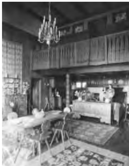
This 1932 photo shows the extensive woodwork that Villaume supplied for the interior of Louis W. Hill's residence in North Oaks. Much of the wood in Hill's "Swiss Chalet" was specially selected and sawed California redwood. Photo courtesy of the Louis W. Hill Papers, James J. Hill Reference Library.
