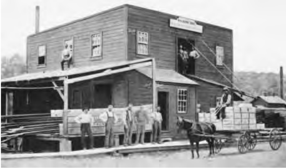
This converted building served as the Villaume brothers' first plant on St. Paul's West Side between 1882 and 1886.
