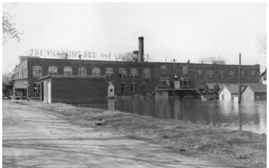
After Mississippi River water from the 1952 flood had started to recede, a photographer was able to show how completely the river had overrun the West Side flats and isolated the Villaume plant.
