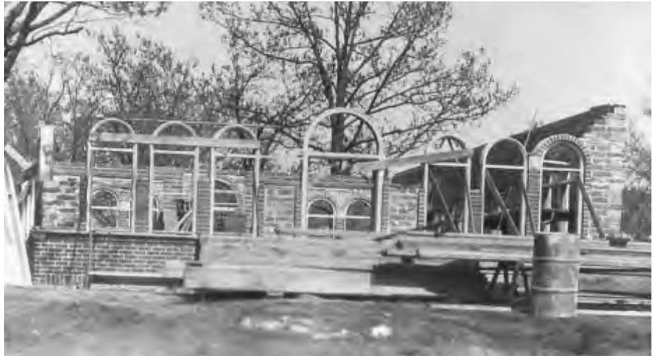
Another photo from May 1929 shows the partially completed pavilion in Newell Park with its distinctive façade of a single entry centered between two sets of three arched windows. Photo courtesy of the St. Paul Parks and Recreation Department.
