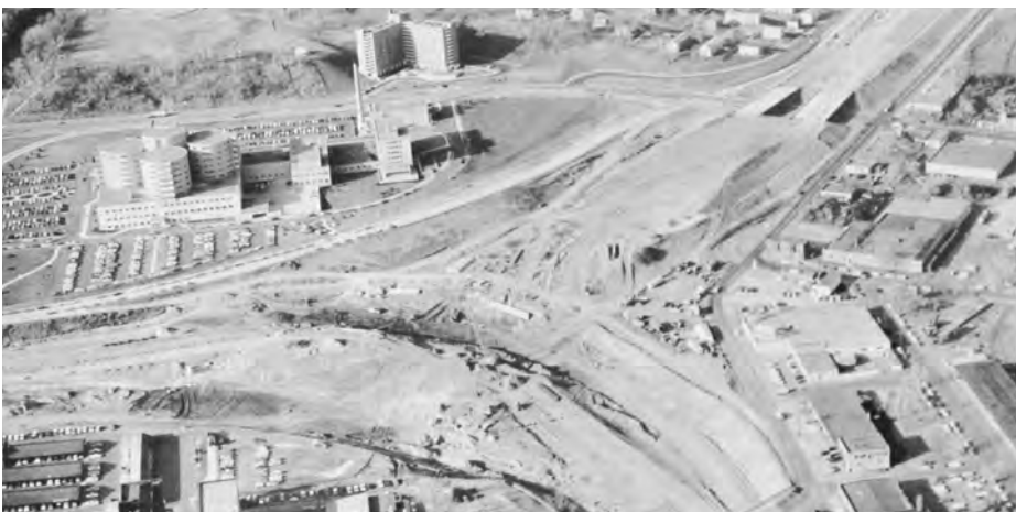
In this 1966 aerial photo, the roadbed for I-94 arches across the bottom of the construction area and the outline for the potential interchange with I-35E runs from the top right toward the center left just below the St. Paul-Ramsey (now Regions) Hospital, located in the top left portion of the area. Photo courtesy of the Minnesota Department of Transportation.
