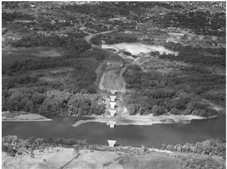
Although the Pleasant Avenue corridor was the area of St. Paul through which planners routed I-35E, the initial construction, seen in this September 1962 aerial photo looking across the Mississippi toward West Seventh Street, required the building of concrete supports for the bridge that would soon cross the river. Photo courtesy of the Minnesota Historical Society.
