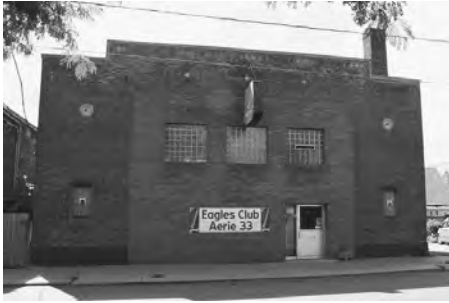
In 1953 Ralph Scalze negotiated the purchase of this building on Maria Avenue as the headquarters for Local No. 20459. Today it's the home of Aerie 33 of the Eagles fraternity. Photo courtesy of Gerald E. Scalze.
