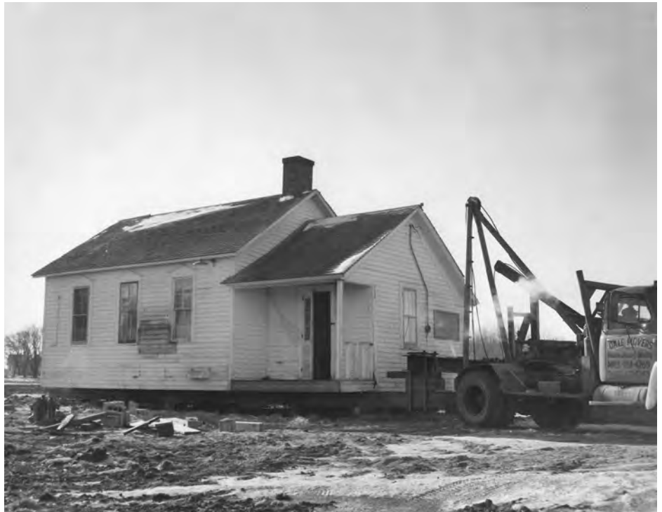
In the mid-1970s RCHS moved the one-room Stoen Schoolhouse from Chippewa County to the Gibbs Museum. Although the schoolhouse took up all the available space on this trailer, the wooden structure was not that difficult to transport roughly 140 miles to its current location in Falcon Heights. Photo courtesy of the Ramsey County Historical Society.
