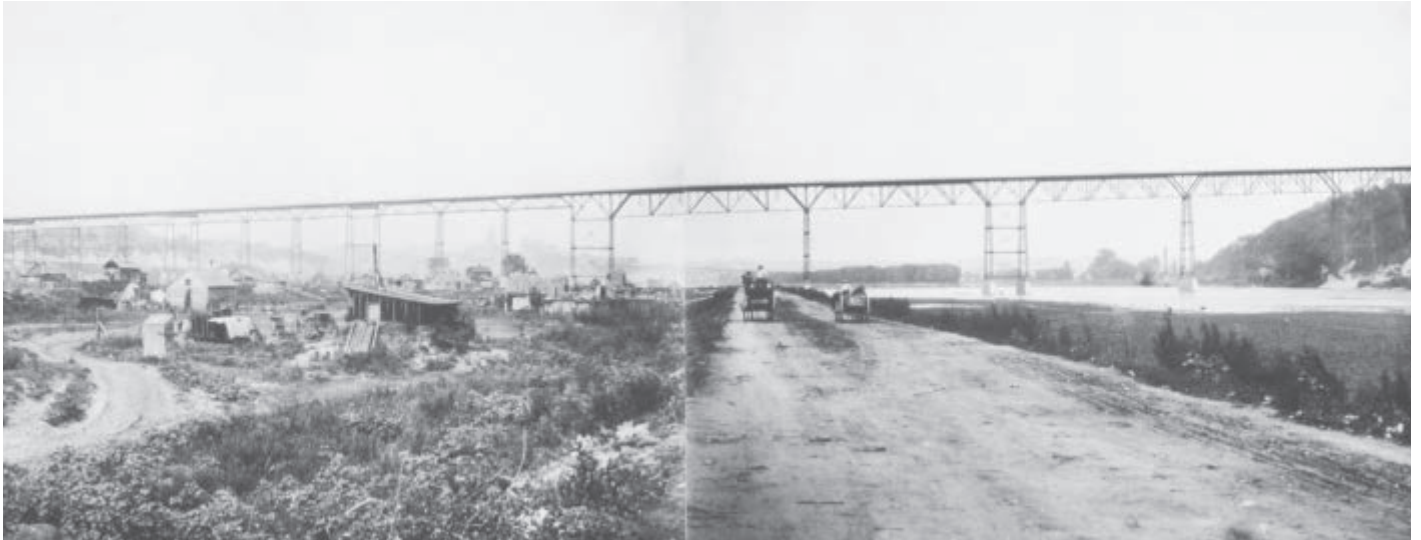
This 1889 photo taken from the Upper Levee flats on the north side of the Mississippi shows how the High Bridge rises at a continuous 4% grade. Photo by the Northwestern Photo Company, courtesy of the Minnesota Historical Society.
