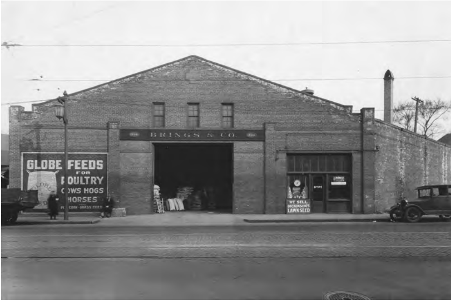
Frank did not carry insurance on the Brings and Company building so the fire resulted in a tragic loss for Frank and his family. With the help of friends and neighbors, however, Frank built a new brick building, seen here in this undated photo, within a year. Photo courtesy of the Kremer Family Collection.
