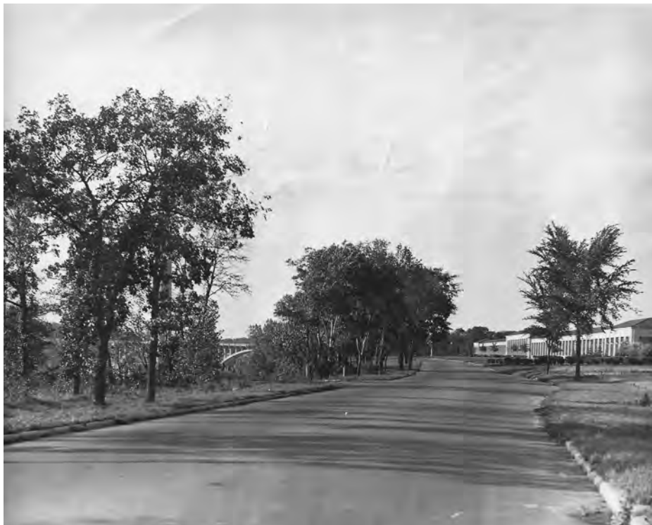
This 1931 photo shows how the Mississippi River Boulevard approached the Ford Assembly Plant from the south. In the distance on the left is the Intercity (Ford) Bridge, which was completed in 1925. Photo courtesy of the St. Paul Parks and Recreation Department.
