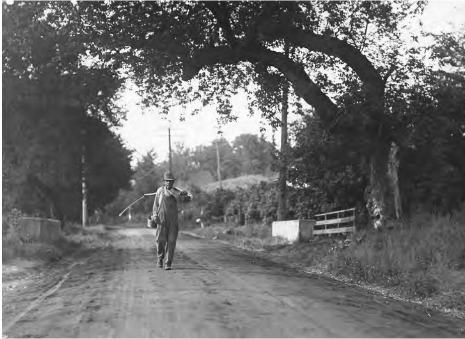
Mississippi River Boulevard before it was graded and widened in the late 1920s. Photo courtesy of the St. Paul Parks and Recreation Department.
