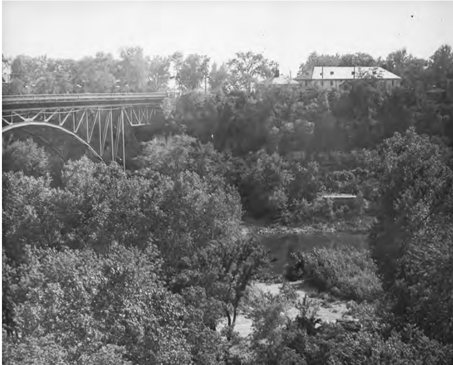
Three bridges have crossed the Mississippi River from West Seventh Street to Fort Snelling over the years. The first bridge was completed in 1880. It was replaced in 1909 with a continuous steel arch truss bridge, seen here from Mississippi River Boulevard looking west toward the fort. The current bridge in this location opened in 1965. Photo courtesy of the St. Paul Parks and Recreation Department.
