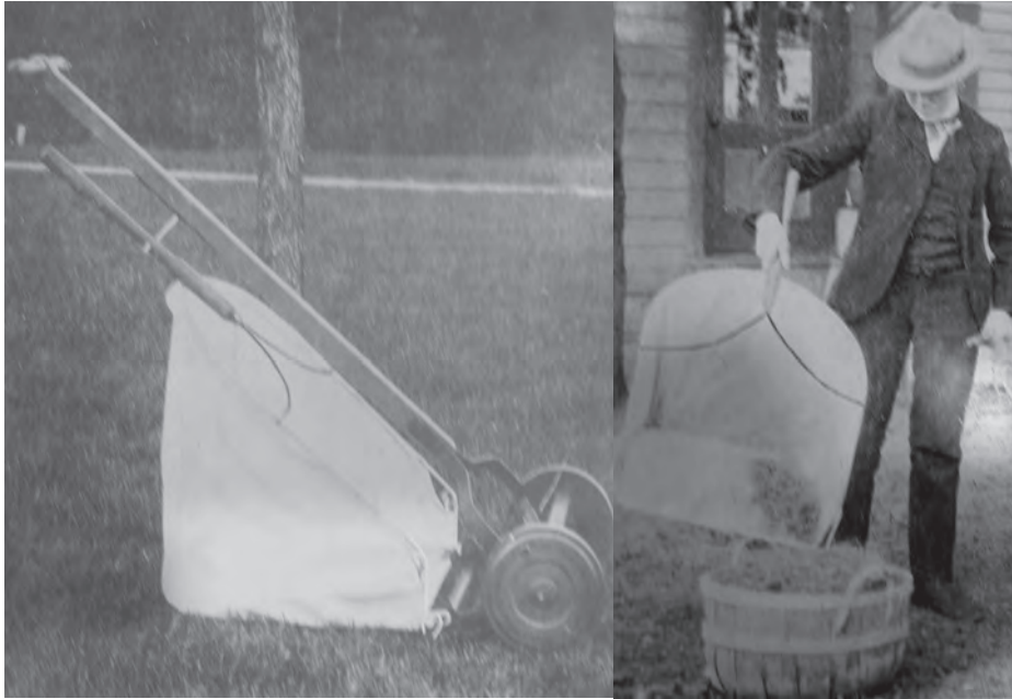
Left, the Easy Emptying Grass Catcher that Boss invented attached to a standard reel, push-type, lawn mower. Right, Boss demonstrating the ease of emptying the grass catcher. Boss Family and Business Collection. Photo courtesy of the Minnesota Historical Society.
