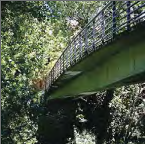
Bridges Over Barriers
