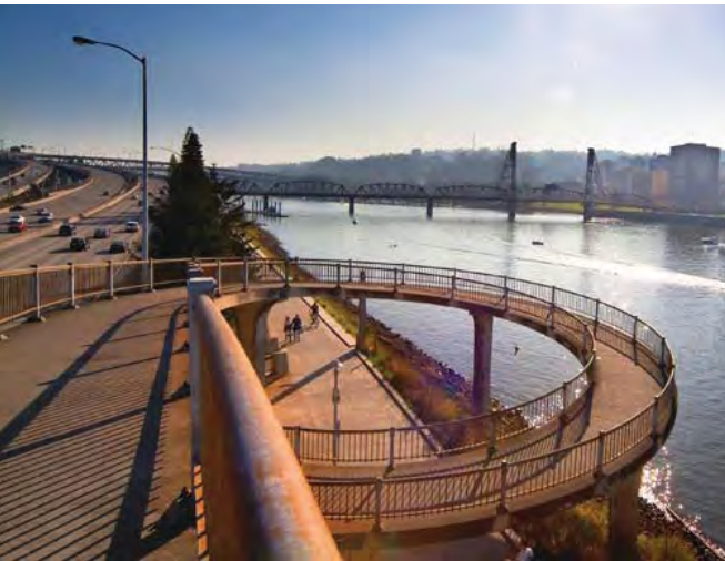
Grade-Separated Crossings: Structures are reserved for roadways with high traffic volumes and speeds, where crossing at a signal is not practical.
