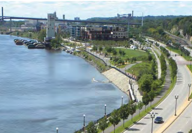
The river’s edge must balance commerce, transportation and redevelopment with recreation and open space.
