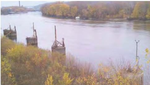
Existing abandoned barge docking facility
