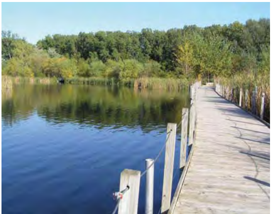
Boardwalks provide access to sensitive ecologies
