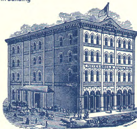
John Wann Building
