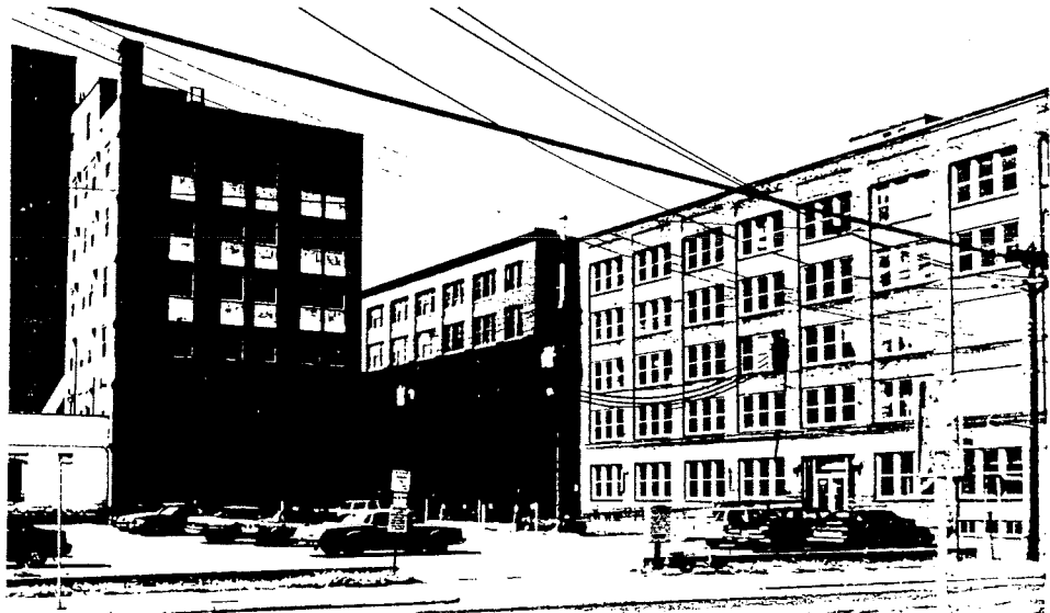
Photo 16 (1989). Looking toward the O'Donnell Shoe Co. Buildings and the McGill-Warner Co. Building from Ninth and Temperance. While these buildings would be considered supportive in the Lowertown District, they are later, different in style, and physically so separated from the district that it is difficult to justify the proposed finger-shaped district expansion to include them.
