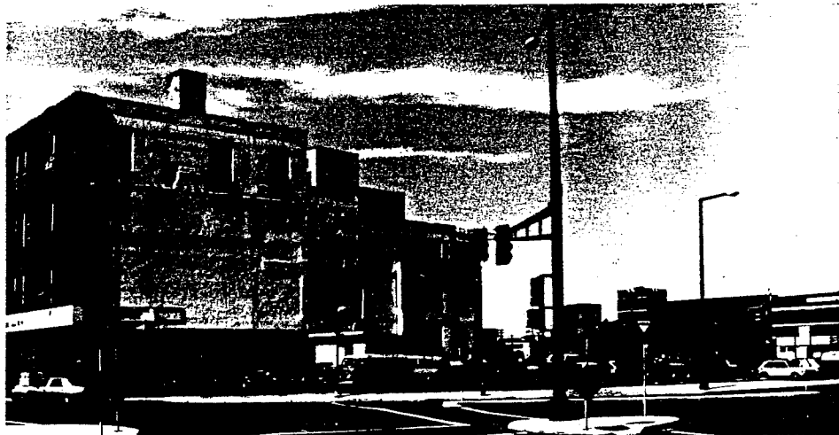
Photo 2 (1989). This is a view of the northeast corner of Seventh and Sibley today, showing the Krahmer Building and all other buildings on the north side of Seventh Street gone and showing a side wall of the City Motor Supply Company Building. This reinforced concrete parking ramp is not associated in use or stylistic detail with the railroad related warehouse and wholesale buildings of Lowertown.
