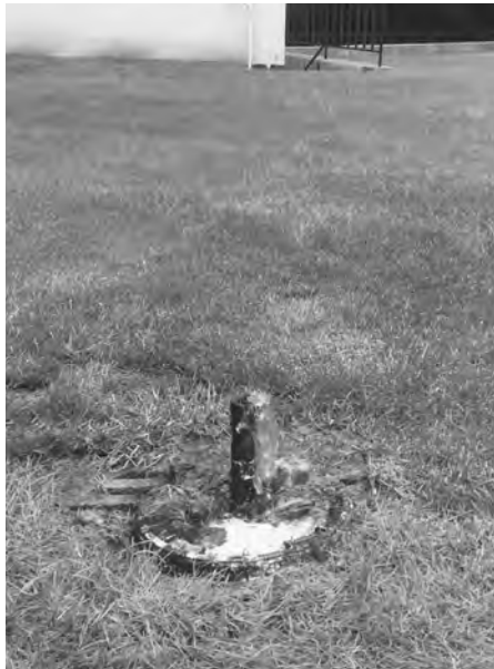
Today the spring bubbles to the surface from an eight-inch pipe installed by the previous owners of the property. Recent measurements indicate the water flow is 3 gallons per minute. Photo courtesy of Greg Brick, Minnesota Department of Natural Resources.
