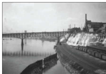
Figure 34. Bluff below Wabasha Street Bridge in ca. 1917 with cribbing (left); Corps of Engineers embankment, 1936, shown during 1951 flood (right).
