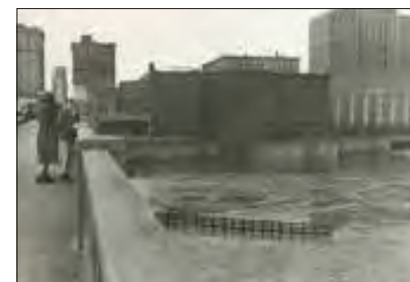
Figure 34. Bluff below Wabasha Street Bridge in ca. 1917 with cribbing (left); Corps of Engineers embankment, 1936, shown during 1951 flood (right).
