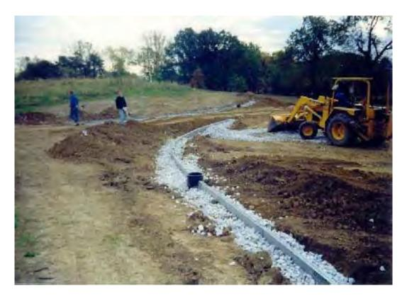
Figure 9.16 Installing a Level Spreader at Coffee Creek Center
