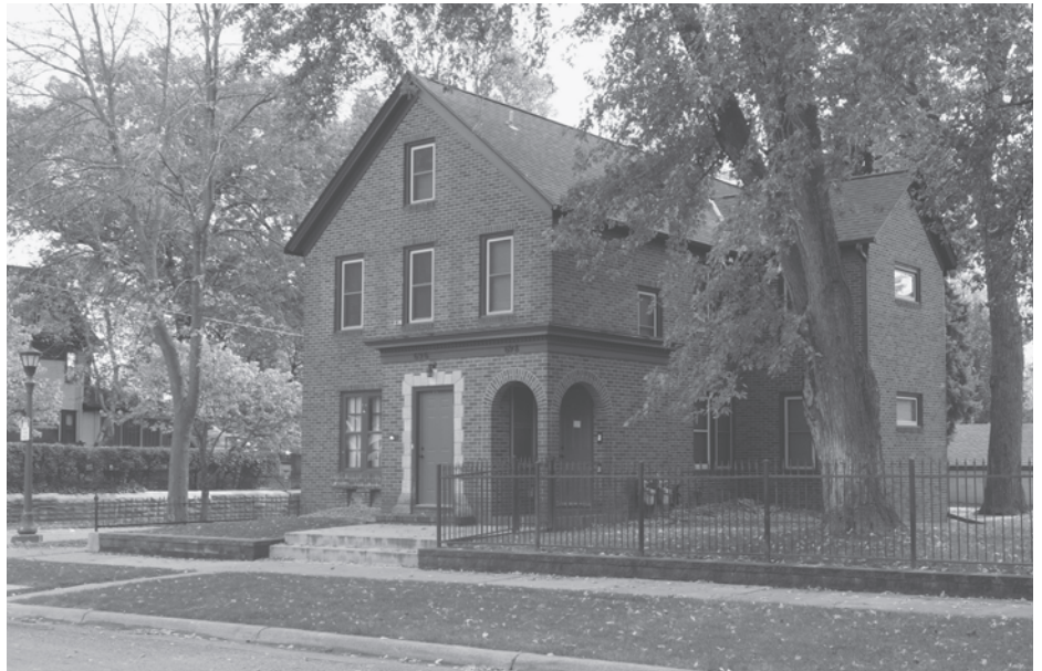
The Gruetzke/Brunson residence, 698 Hawthorne in St. Paul, as it appears today. Emma spent her entire childhood and most of her adult life in this house. Built by her father in 1887, the original clapboard structure was expanded and remodeled several times. In 1933, Emma added brick veneer and an entry vestibule with two separate entrances. Most of the divided-light windows have since been replaced. Photo courtesy of Diane Trout-Oertel.
