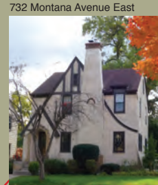
732 Montana Avenue East
