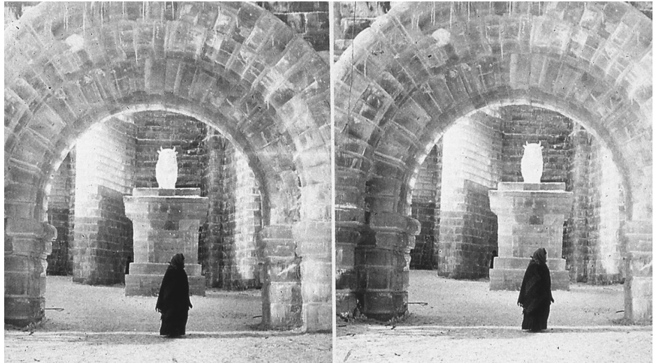
This stereoscopic view of the main entrance to the 1887 ice palace showcases the skill of St. Paul's stonemasons, which is evident in the high degree of architectural detailing and joinery that was used in the construction of the archway. Henry Hamilton Bennett photo. Photo courtesy of the Minnesota Historical Society.
