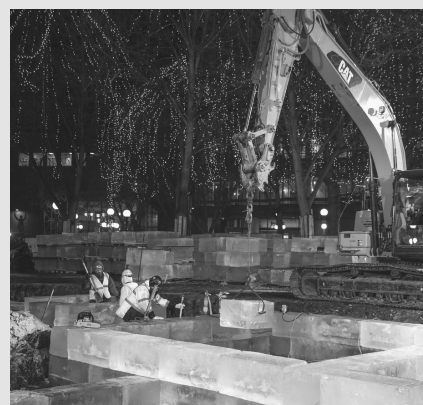
Large cranes are essential tools in the hoisting and maneuvering of the 400-pound ice blocks that are used in the construction of the 2018 Ecolab Ice Palace. In the rear of this nighttime photo, lights illuminate the lobby of the Ordway Center for the Performing Arts. Darrin Johnson photo. Photo courtesy of Darrin Johnson and the Saint Paul Winter Carnival.
