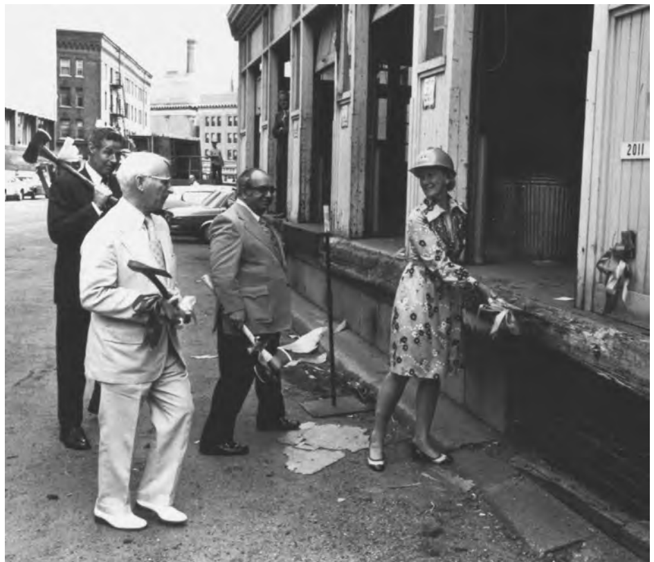
Betty Musser, right, Frank Marzitelli, center, Carl Drake, far left, and Ron Hubbs wield axes in a symbolic demolition of a portion of the loading dock used by the former Post Office prior to the beginning of the renovation of the building in 1975. Betty Musser represented Minnesota Landmarks, Frank Marzitelli represented the Saint Paul Port Authority, and Carl Drake and Ron Hubbs represented the St. Paul Companies (now Travelers), which supported restoring the Courts Building. Photo courtesy of Minnesota Landmarks.
