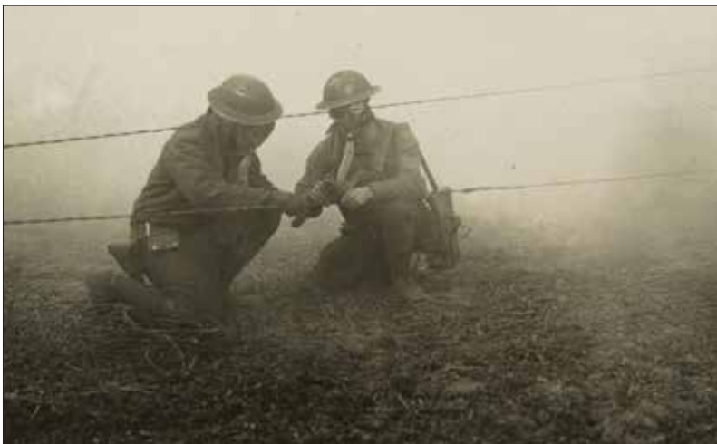
Trapped in a haze of gas on the front lines in France, two American soldiers repair phone lines while wearing gas masks. Photo courtesy of the Smithsonian Institution, Washington, D.C.
