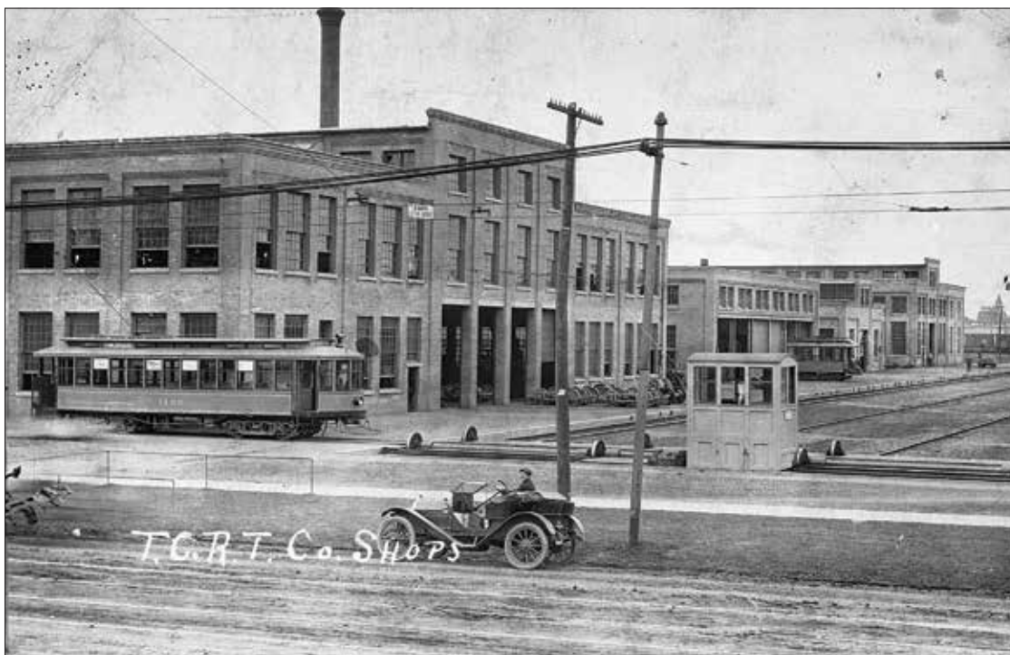
This 1910 view looks east from Snelling Avenue, showing TCRT's machine shop in the foreground and a row of other shop buildings running parallel to the transfer table. The streetcar will move on the transfer table and be shunted to one of the shop buildings. Forty years later, the automobile will make all of this irrelevant. Photo courtesy of the Minnesota Historical Society.
