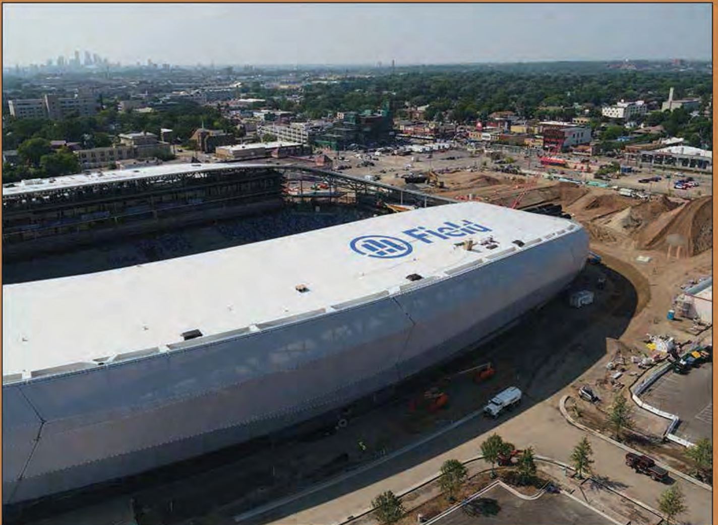
The Minnesota United Football Club expects Allianz Field, its new soccer stadium, to open for play in early 2019. The capacity of this soccer-specific facility is more than 19,000. This aerial photo from August 2018 shows that much of the exterior of the stadium has been completed on the site that was once the TCRT's Snelling Avenue repair facility. University Avenue and the nearby station on Metro Transit's Green Line can be seen on the right. Snelling Avenue runs north-south on the far side of the stadium. In the distance is the Minneapolis skyline. Photo courtesy of the M. A. Mortenson Company.
