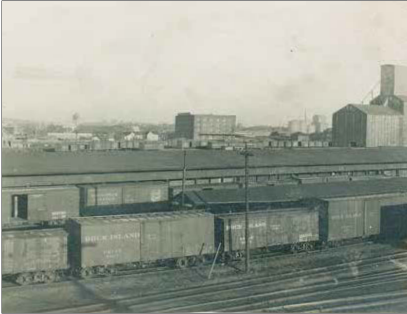
The Minnesota Transfer Railway Company yards in 1917. Today, the location of the Transfer's original boundaries includes the BNSF rail tracks adjacent to the Pierce Butler Route on the north; Fairview Avenue on the east; St. Anthony Avenue on the south; and Cleveland-Vandalia Avenues on the west. Photo originally from Midway Chamber of Commerce. Courtesy of the Ramsey County Historical Society.
