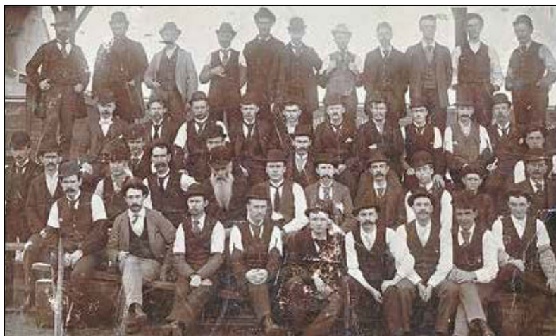
Hundreds of employees, working as clerks, engineers, veterinarians, agents, mechanics, and in many other roles, helped the Minnesota Transfer Railway run smoothly (March 12, 1893). Back row (L-R): 2. Jack Gallagher, customs collector; 3. Mr. Ackerman, clerk; 4. Mr. Sanders, cashier and later, agent; 6. M. J. Dooley, chief clerk and later, superintendent; 10. Mr. Briggs, cashier; 11. Phil Donnelly, clerk. Fourth row (L-R): 2. M. A. Gilman, clerk and later, agent and local art, Detroit Lakes; 4. Mr. Chapman, cashier; 5. Dan Hanrahan, clerk; 8. Mike Fanghnan, clerk. Third row (L-R): 1. B. E. Graves, foreman; 3. H. L. Burrill, agent; 4. Joe N. Deller, clerk and later, traffic manager for U.S. Steel, Duluth. Second row (L-R): 1. Roger Reilly, cashier (Northern Pacific and Minneapolis & St. Louis Railway); 2. L. A. Baker, clerk and later, agent with Northern Pacific, Aitkin; 3. Mr. Quigley, clerk and later, chief clerk; 6. Dave Mulreim, clerk and later, agent at Grand Forks, St. Paul, and Minneapolis; 8. Mike Readon, clerk; 10. Chas Segerstrow, messenger law at Los Angeles; 11. J. F. (Doc) Jones, inspector. Front row (L-R): 3. Harry Donnelly, telegraph operator; 5. Mr. S. Schneider, clerk and later, chief clerk; 7. Jack Stark, cashier. Courtesy of the Ramsey County Historical Society.
