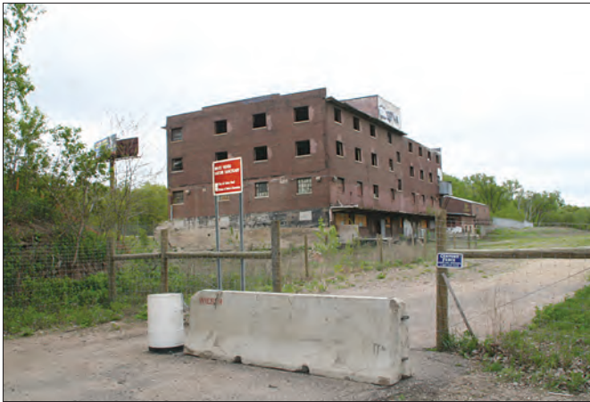
This 1914 Standard Oil building was an empty, abandoned eyesore. The city purchased it in 2009. For a time, LPCP had hoped to remodel the structure as an education center at the edge of Bruce Vento Nature Sanctuary. Courtesy of Dan McGuiness.
